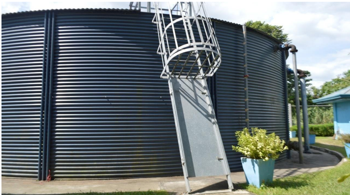
Magsaysay Reservoir Compound, Brgy. Magsaysay, Kidapawan City
